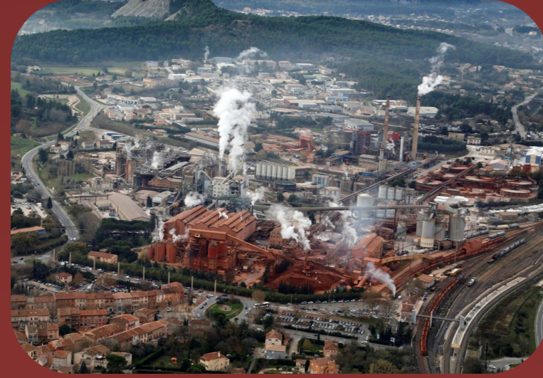
Alteo Gardanne plant
