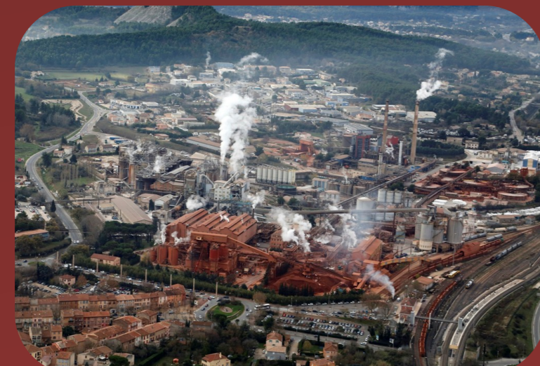
Alteo Gardanne plant
