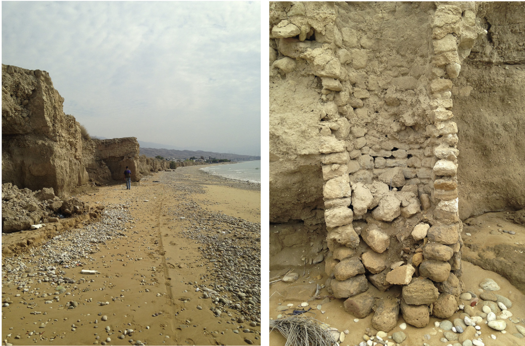
Fig. 9. Photographs of the coastal erosion at the base of Siraf's old city walls (Group 3 transects).
