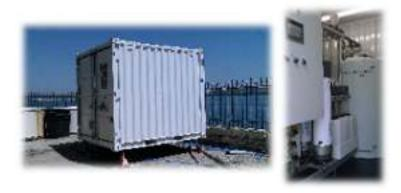
Figure 1. UF pilot plant [2 industrial modules 84m2, MWCO = 100kDa]
