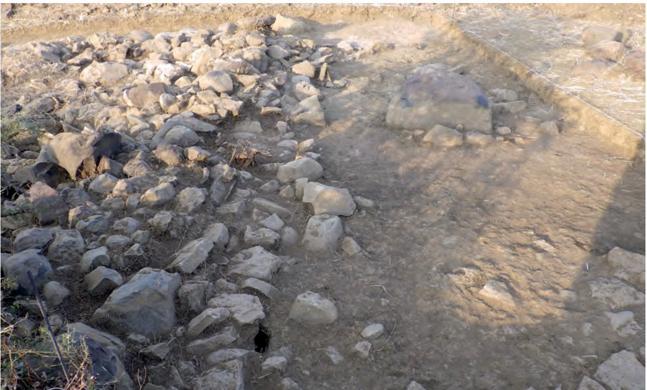
Fig. 94: Walls 3004 and 3006 looking north. Note the hole corresponding to the foundation trench of Wall 3004
