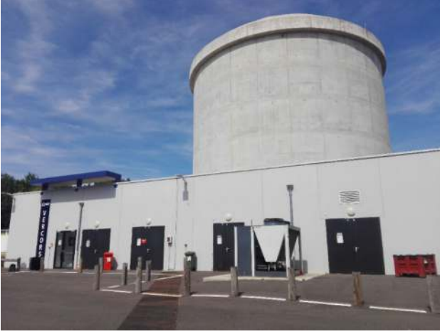
Fig. 1 Photograph of Vercors building mock-up
