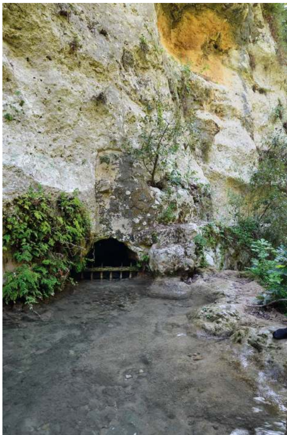
Fig. 4 The Calcinara water intake.
