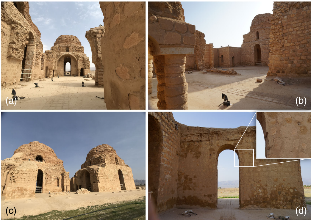
FIGURE 2 The Sarvestan monument from different angles. (a) Looking to the second dome in NNE-direction through the eastern hall. (b) Looking to the internal courtyard from the opening of the western eyvan . The western columned hall is located on the left. (c) a view to the north showing the two main domes as well as part of the eastern columned hall. (d) the southern wall of the western eyvan with the position of one of the oldest wood samples (S39)
