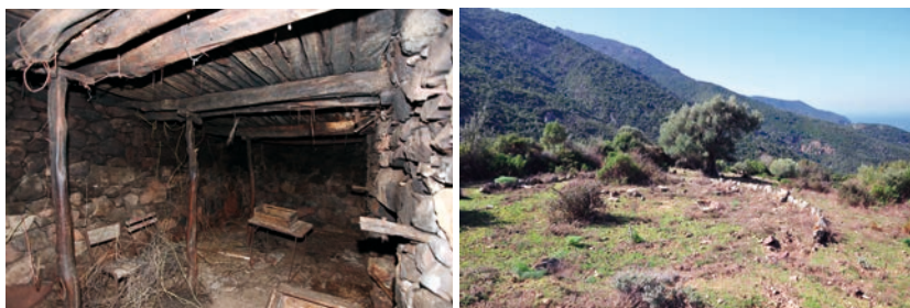
Figure 6. Left. A shepherd's stone hut ('stazzu') at L'Elbu. Note the pillars and the roof made of juniper wood ( Juniperus oxycedrus ). Right. A threshing floor ('aghja') at L'Elbu. Photos © Jean-Marie Dominici.
